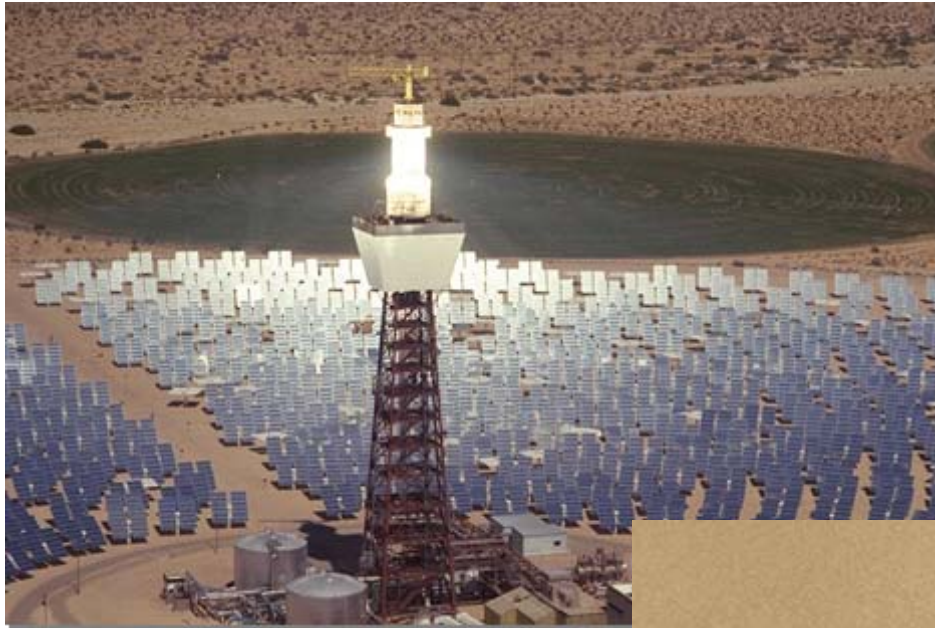
Solar II Solar Central Receiver
