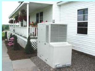
100 kW, 15 kWh li-ion battery for UPS applications
