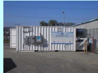
100 kW, 15 kWh li-ion battery for UPS applications
