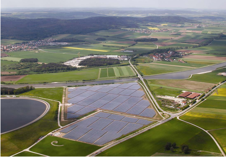
SunPower Systems' 10-MWp large field installation in Bavaria
