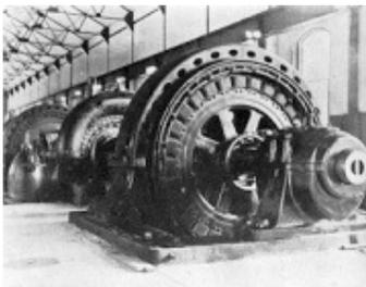
*The DeCew Falls Hydro-Electric Development was a pioneering project in the generation and transmission of electrical energy at higher voltages and at greater distances in Canada. On 25 August 1898 this station transmitted power at 22,500 Volts, 66 2/3 Hz, two-phase, a distance of 56 km to Hamilton, Ontario.*
