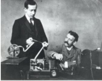
*At Signal Hill on December 12, 1901, Guglielmo Marconi and his assistant, George Kemp, confirmed the reception of the first transatlantic radio signals. With a telephone receiver and a wire antenna kept aloft by a kite, they heard Morse code for the letter "S" transmitted from Poldhu, Cornwall. Their experiments showed that radio signals extended far beyond the horizon, giving radio a new global dimension for communication in the twentieth century.*
