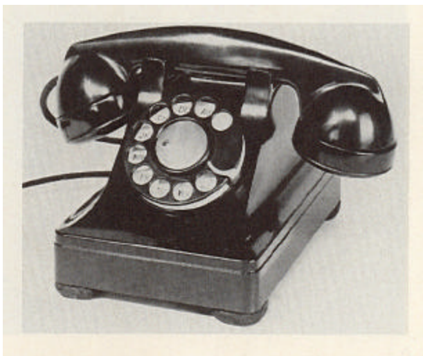
1937 desk telephone with bell concealed in base. Photo courtesy of Bell Canada Telephone Historical Collection.
