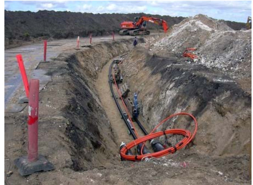
Cross-section of Cable Trench Tebbestrup – Hornbæk
