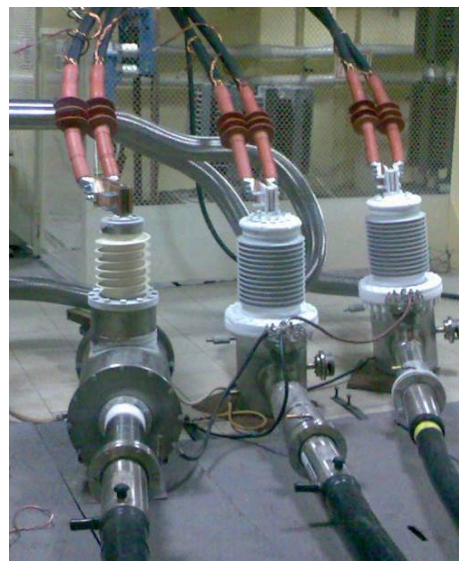
Fig. 2. Two types of current leads connected to the cryostats and electrical system.
