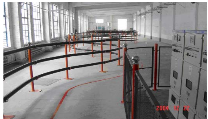
Fig. 16. The installation of the 75 m 10.5 kV/1.5 kA HTS power cable
