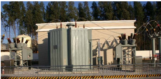
Fig. 18. The installation of 35 kV/90 MVA SISFCL.
