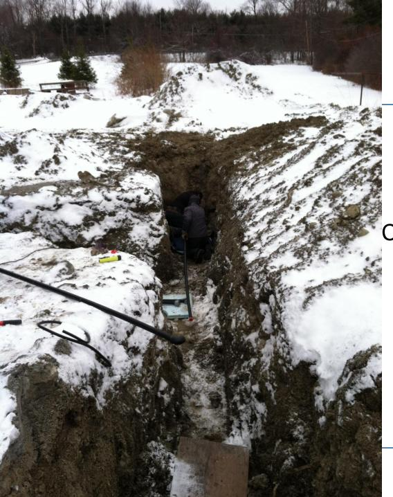
Connections via heat fusion in process
